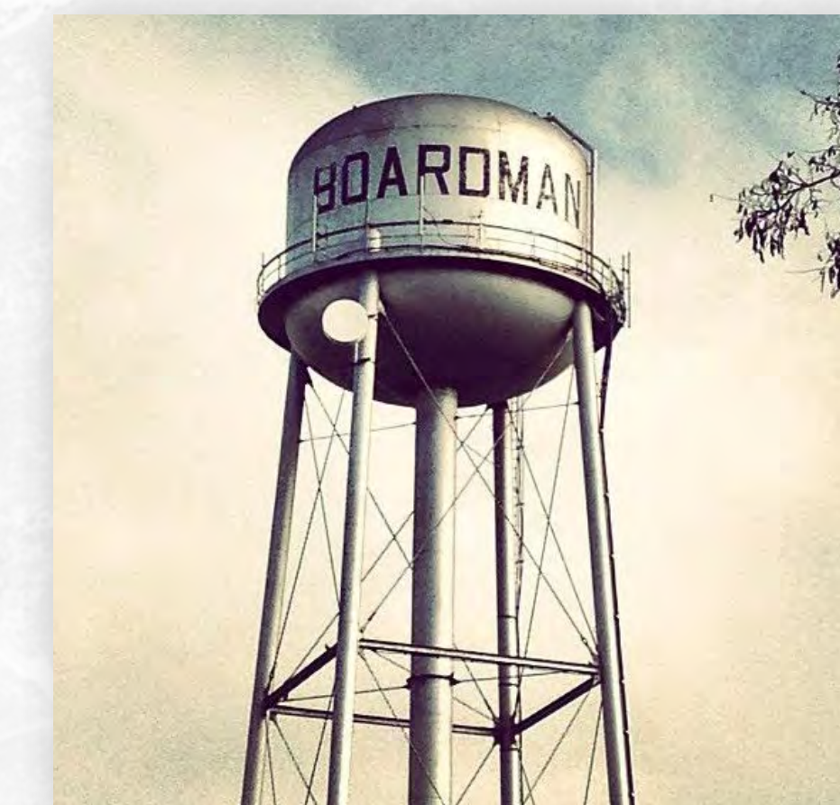
Original Boardman water tower. Torre de agua original de Boardman.
