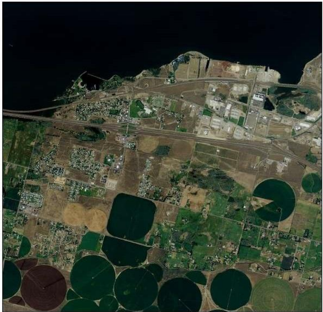
Figure 2-3 Aerial view of Boardman, Oregon
