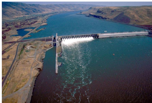
Figure 4: Photo of the John Day Dam
