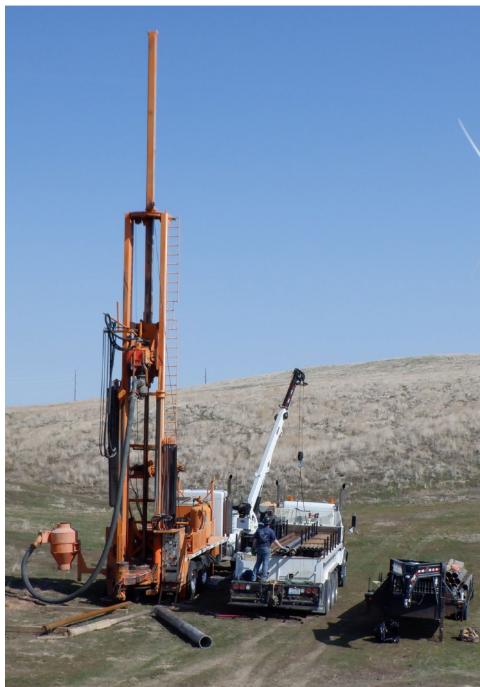
Well drilling (at Farm 4) for Port of Morrow
