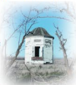
Pump house for water well at Traveler Rest Area. Installed by Sam Boardman on original highway.
