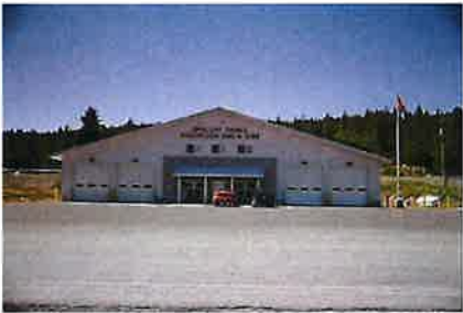
Tribal Fire Station
