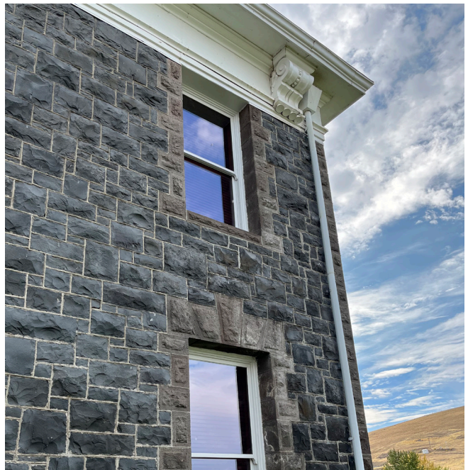
Northwest corner where crack was repaired
