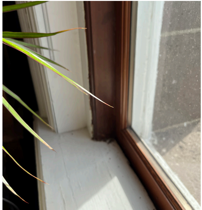
Typical replacement sash
