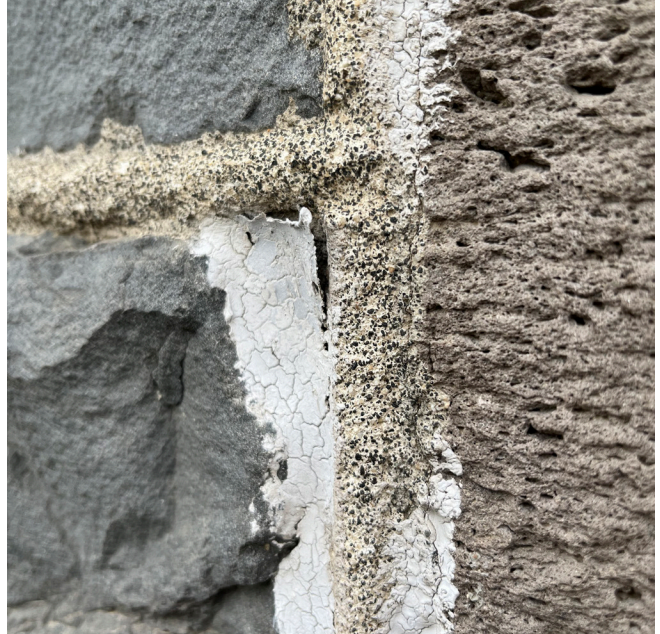
Close-up view of caulking
