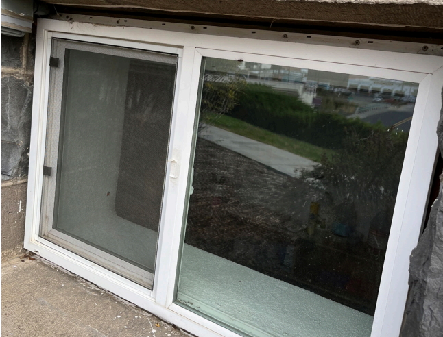
Vinyl replacement window at basement
