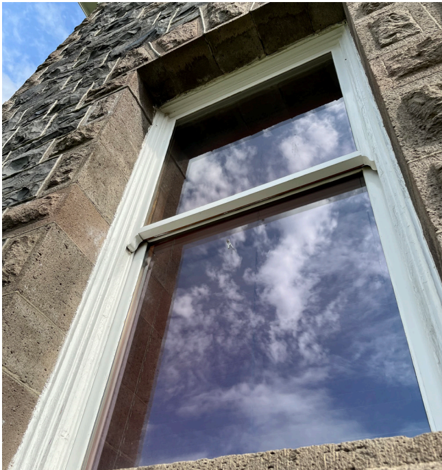
Exterior view of typical window
