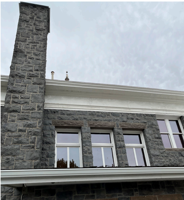
Chimney at east wall
