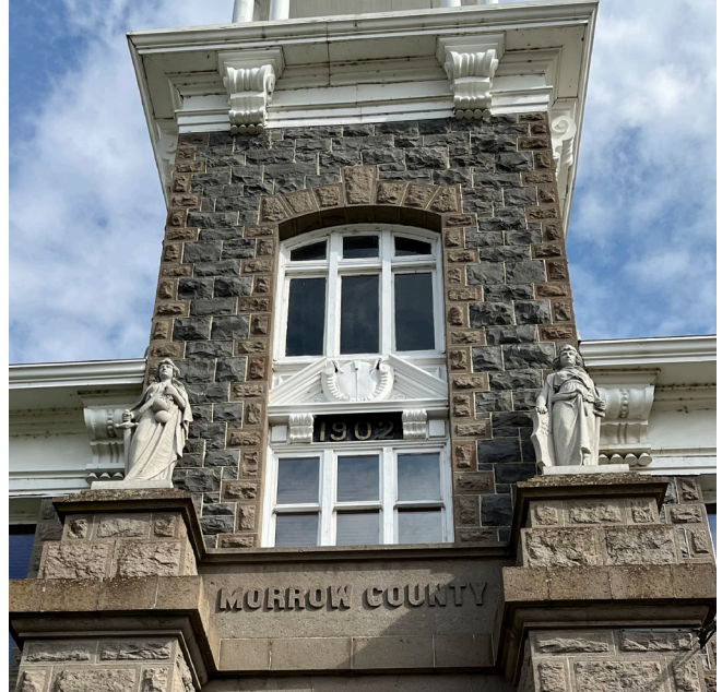
Historic wood windows at bell tower
