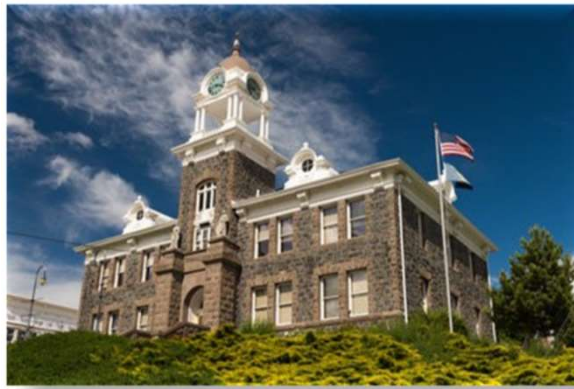
Morrow County COURTHOUSE Heppner, OR
