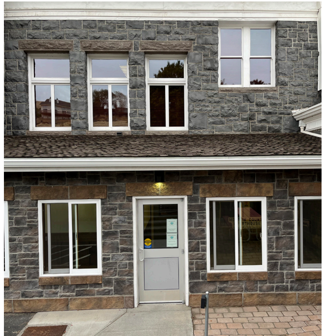
Entry Vestibule at east face of building.
