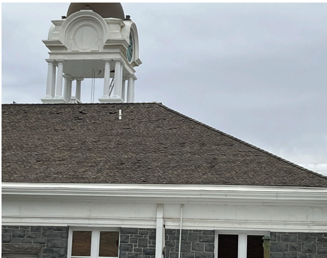
Cedar shake shingle roof
