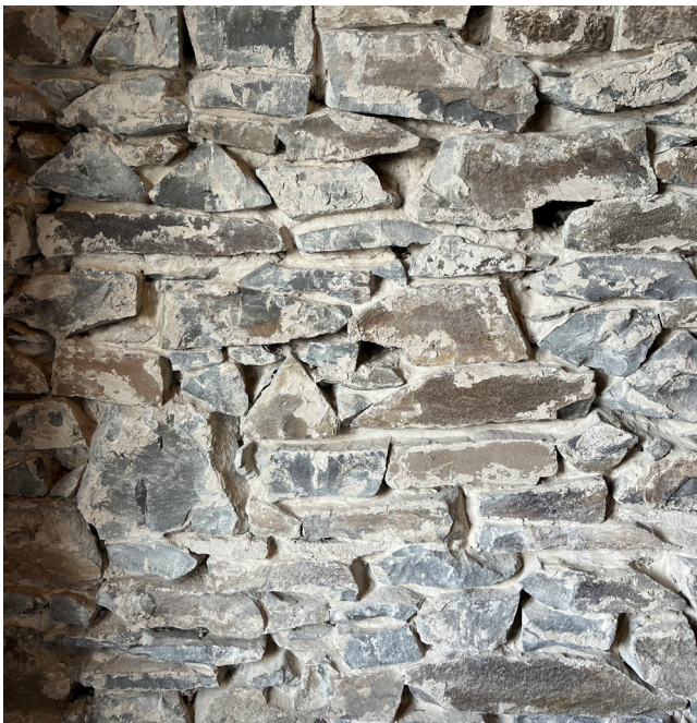
Stone wall at bell tower - mortar removal in process
