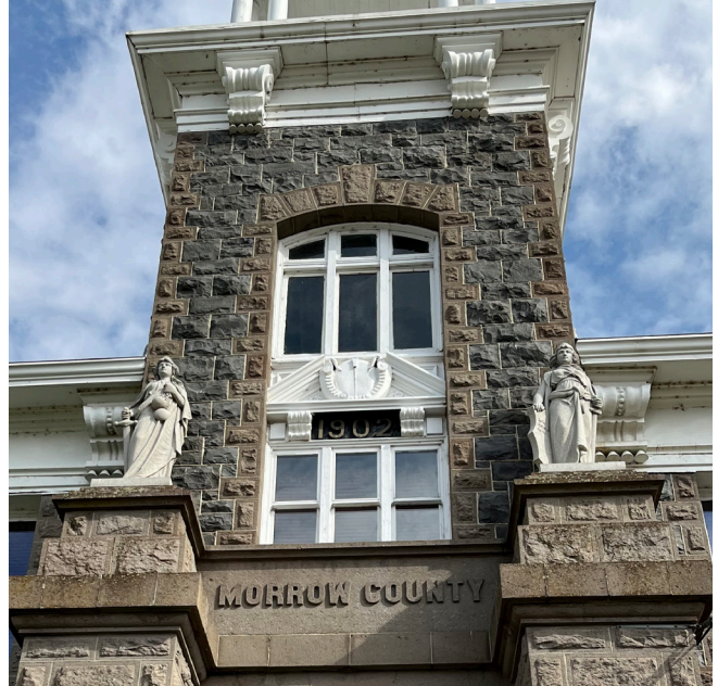
Historic wood windows at bell tower
