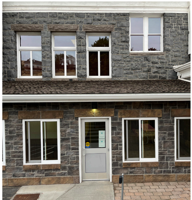
Entry Vestibule at east face of building.
