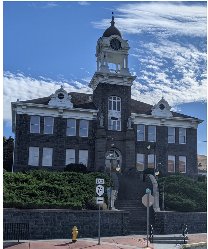
Primary elevation with historic main entry and stone staircase
