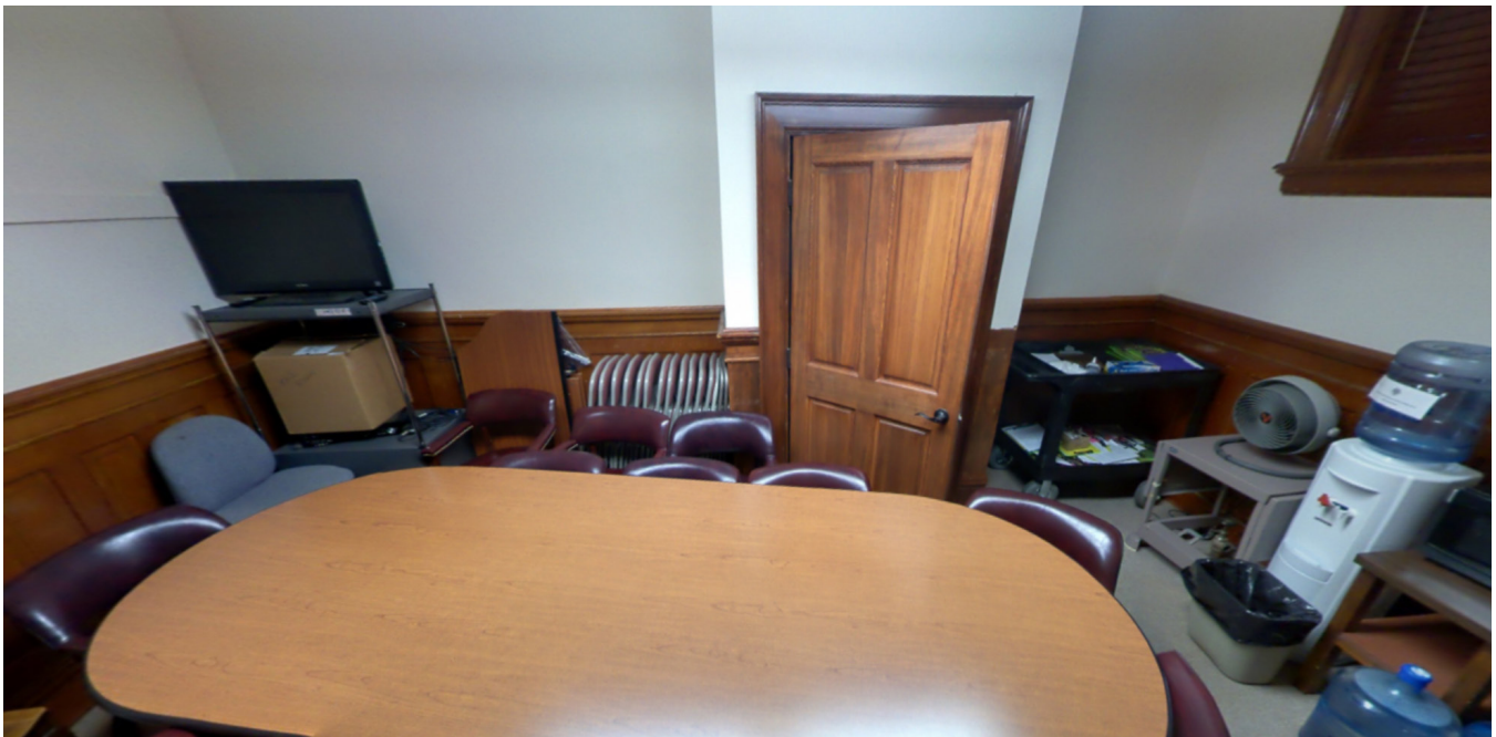
Jury deliberation room directly adjacent to the courtroom with closed for clock cabling.
