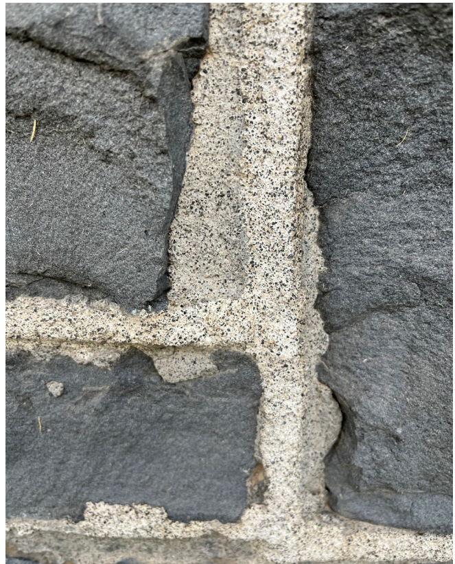
Beaded mortar joint profile
