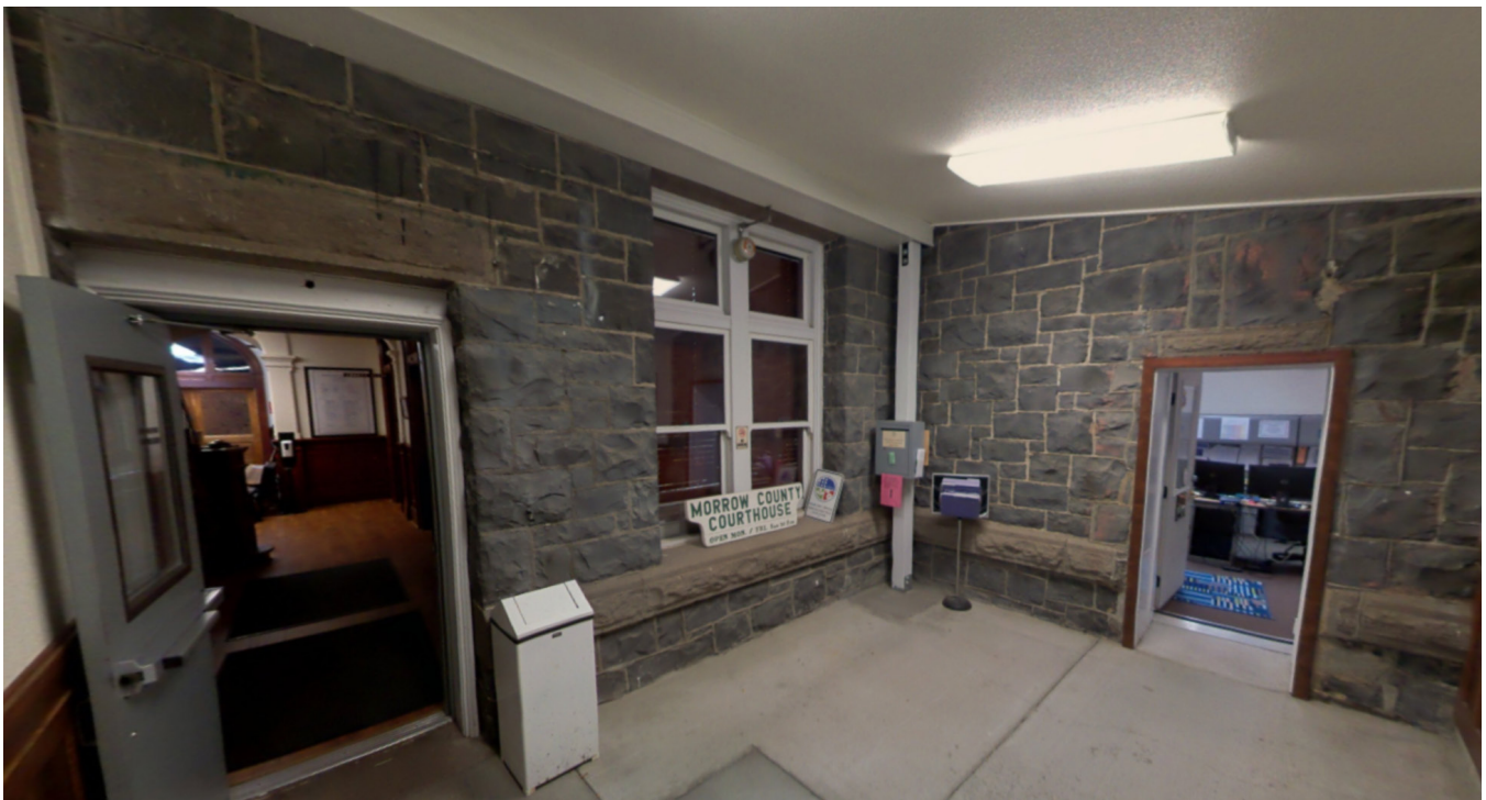
First floor entry vestibule area with door into courthouse on the left and access to Victim Services on the right.
