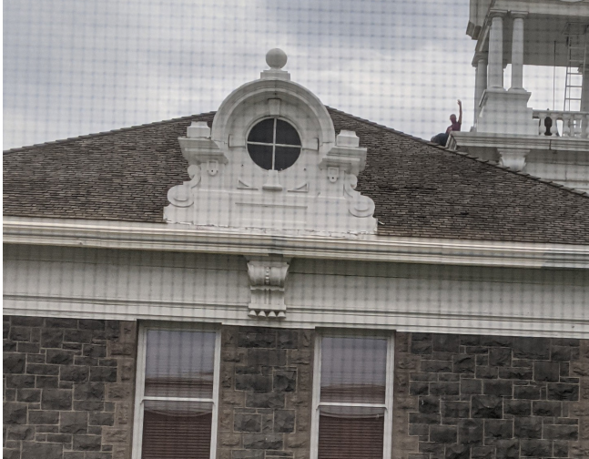
Typical sheet metal dormer
