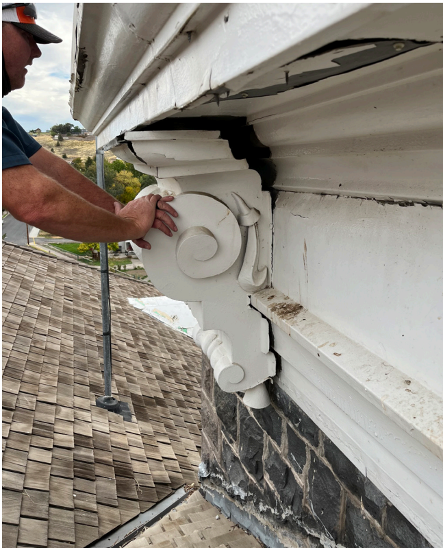
Separating bracket under clock tower
