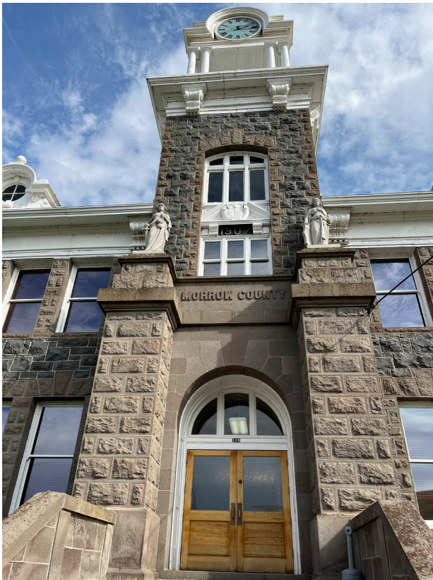
Clock tower with historic main entry below.
