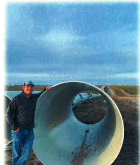
J.R. Cook, NOWA Director, touring a section of the East Project Pipeline (spring/2020)
