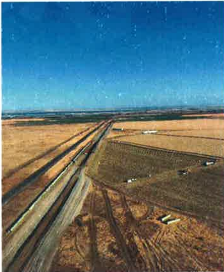
West Project pipeline construction, 2020
