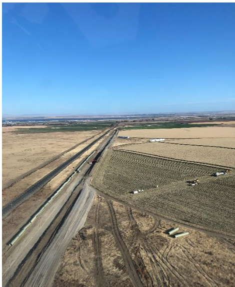
West Project pipeline construction, 2020
