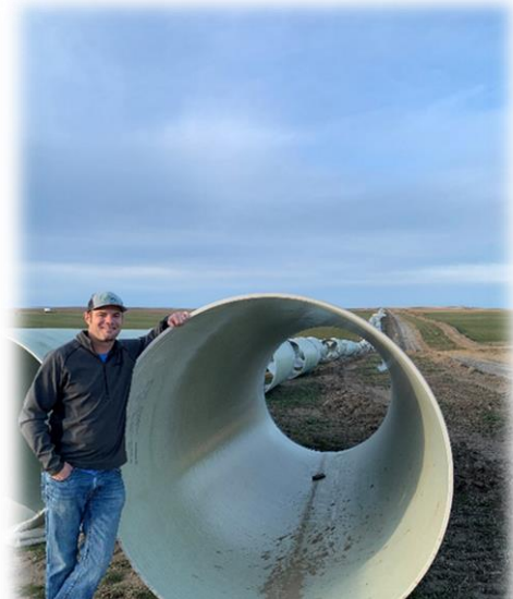
J.R. Cook, NOWA Director, touring a section of the East Project Pipeline (spring/2020)
