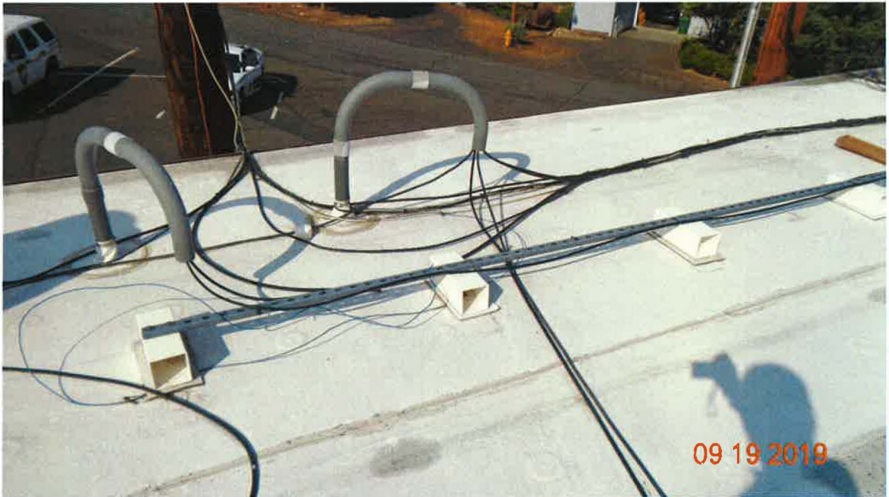
Photo 21: #8 AWG Conductor Bonding the Antenna to SBB#2 in the Equipment Room
