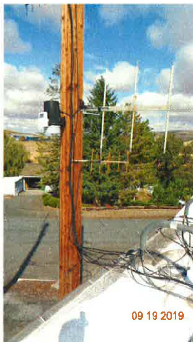
Photo 16: North Side Wooden Pole
