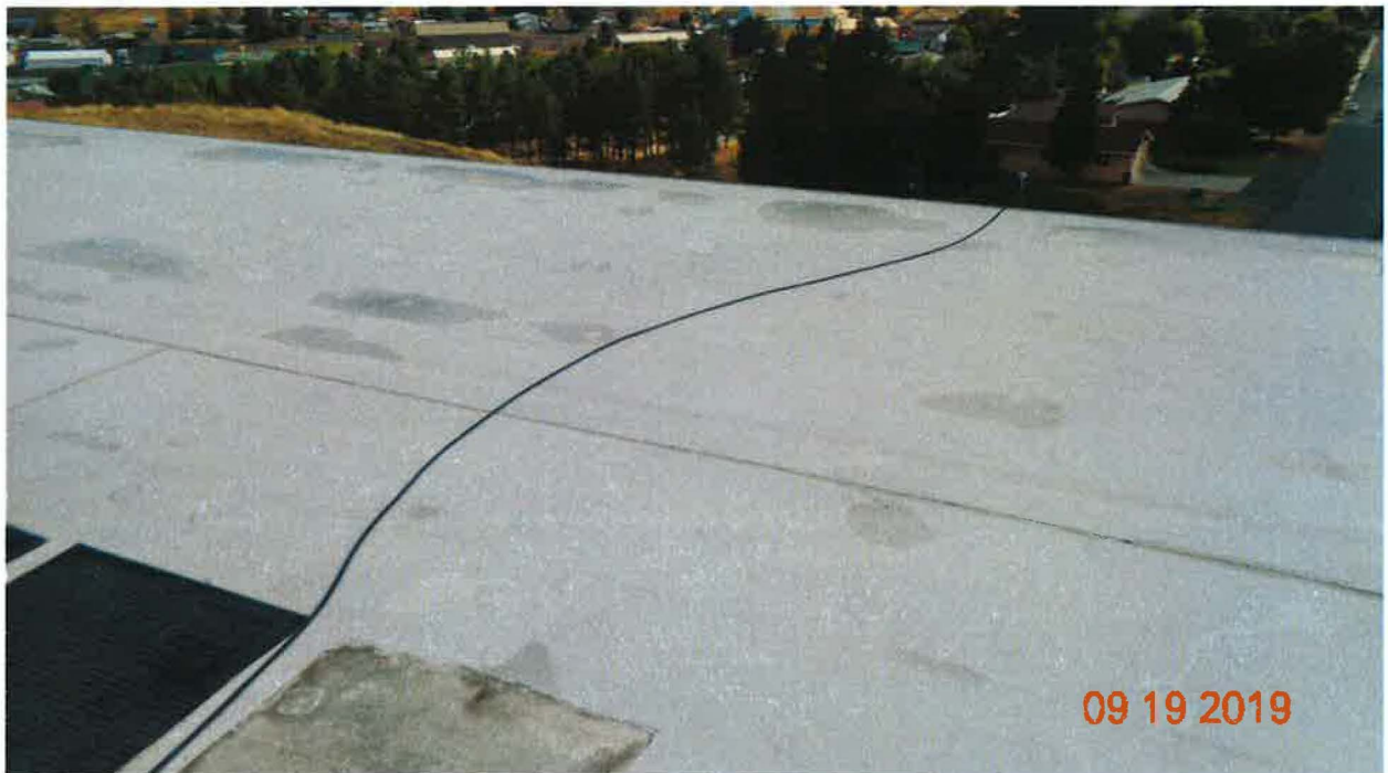
Photo 22: Cable from the HAM Antenna
