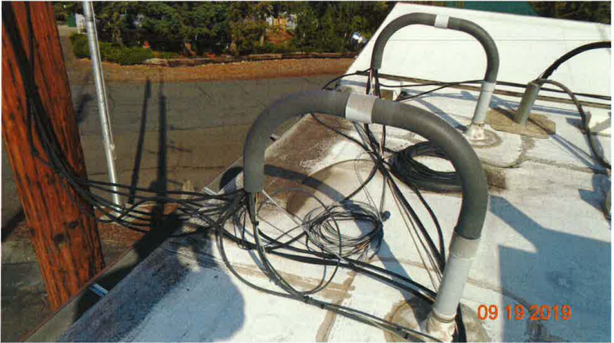
Photo 17: North Side Wooden Pole
