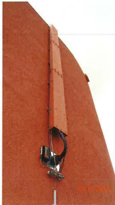
Photo 25: The Existing EGB on the North Side of the Building
