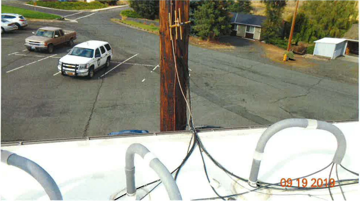
Photo 19: South Side Wooden Pole
