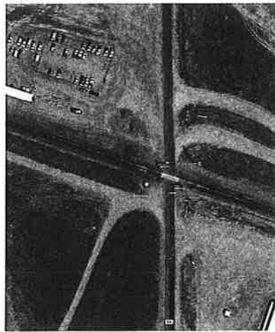
Figure 5: At-Grade UPRR Crossing
